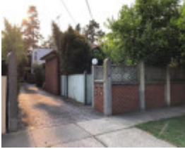
1/80 Repton Road, Malvern East
