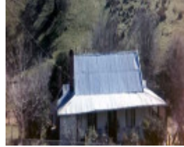
B3568 Maryvale Farm House Leneva West
