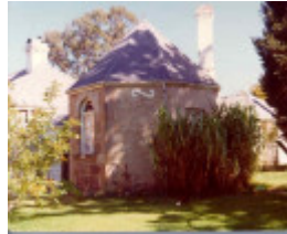
Adelaide Vale octagonal room
