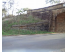
B3602 Blackjack Road Rail Bridge
