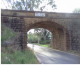
B3602 Blackjack Road Rail bridge
