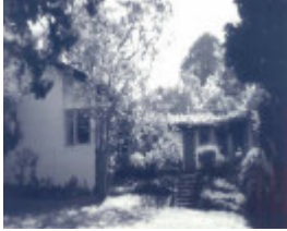
B3818 South Wing & Connecting Gallery
