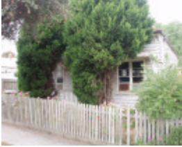
1 Fenwick St South, Geelong
