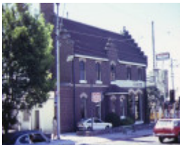
former es&a bank camberwell front view feb1982
