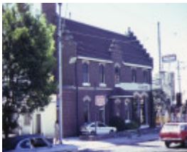
former es&a bank camberwell front view feb1982
