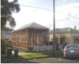
88 Garden Street, Geelong East
