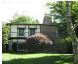
view of house from north 2011
