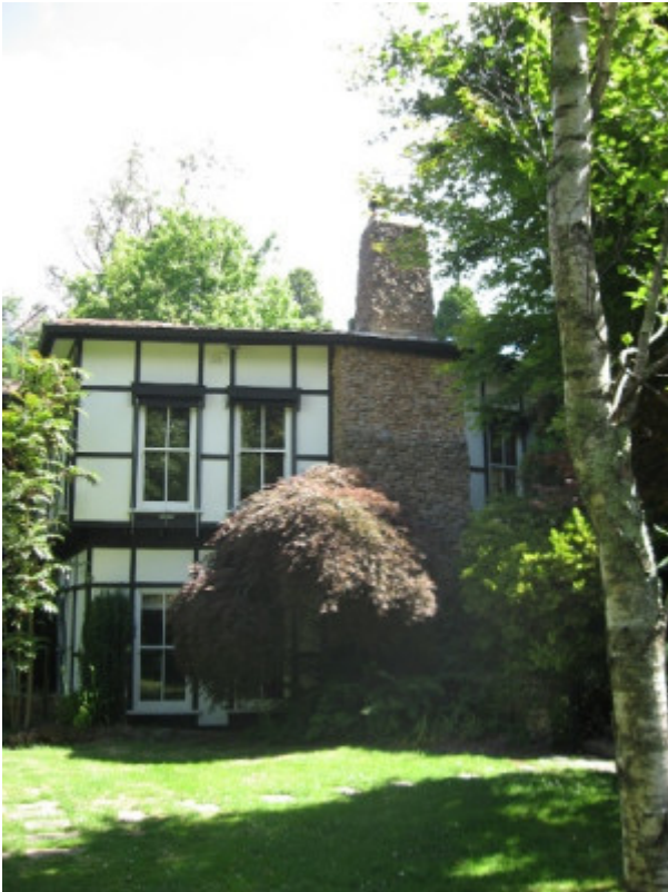
view of house from north 2011
