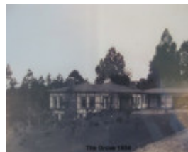
View from driveway 1934
