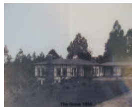
View from driveway 1934
