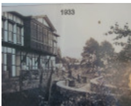
Garden under construction 1933
