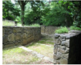
stone walls and steps 2011
