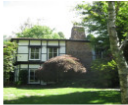
view of house from north 2011
