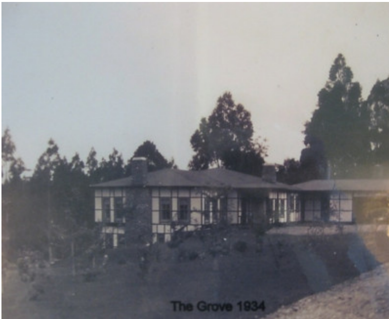
View from driveway 1934
