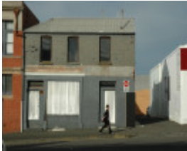
55 Gheringhap Street, Geelong
