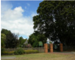
PROV H2214 Portland B G Main entrance gates
