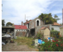
Brick Workshop, west facade
