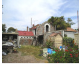
Brick Workshop, west facade
