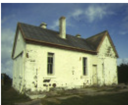
cape otway lightstation signal atation front view aug1996
