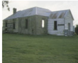
1 former holy trinity anglican church school merrawarp road ceres front view
