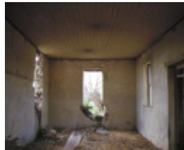
former holy trinity anglican church school merrarp road seres interior
