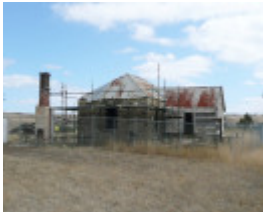
FORMER HOLY TRINITY ANGLICAN CHURCH SCHOOL SOHE 2008
