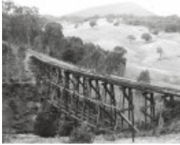
Cudgewa Line Trestle Bridge
