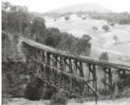
Cudgewa Line Trestle Bridge
