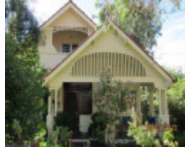
21 Linton Street, Toora Street Precinct
