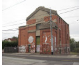
Ascot Vale Substation
