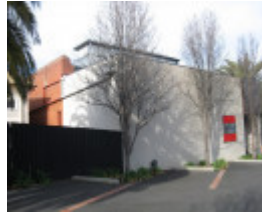
Elsternwick substation rear view
