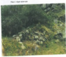
Warby Falls Upper Stone Weir
