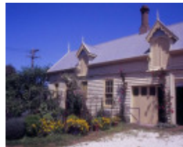
belleville ryrie street geelong stables she project 2004
