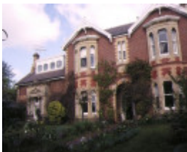
h01188 bellville ryrie street geelong front view aug1995
