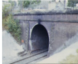
1 railway tunnel geelong colac line geelong front view apr1997
