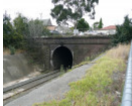
RAILWAY TUNNEL SOHE 2008
