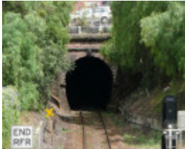
RAILWAY TUNNEL SOHE 2008
