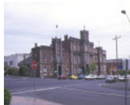
1 gordon technical college geelong front view dec1993
