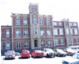
h01019 gordon technical college fenwick street geelong bldga administration bldg she project 2004
