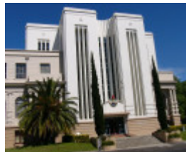
h01019 gordon technical college fenwick street geelong bldg t1 textile college she project 2004
