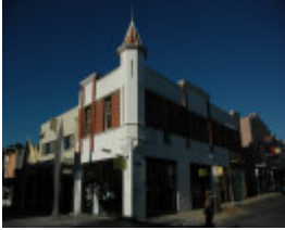
Shop - 80 Lt Malop Street, Geelong
