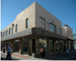
SHop - 87 Lt Malop Street, Geelong
