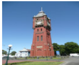
FINLAY AVENUE OF ELMS, MANIFOLD CLOCK TOWER AND PUBLIC MONUMENT PRECINCT SOHE 2008
