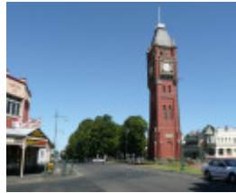
FINLAY AVENUE OF ELMS, MANIFOLD CLOCK TOWER AND PUBLIC MONUMENT PRECINCT SOHE 2008
