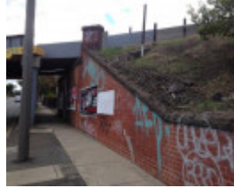
Rail over road bridge Ascot Vale Road
