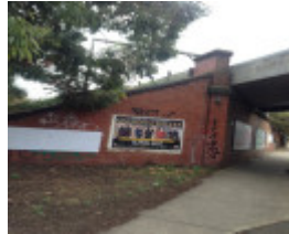
Rail over road bridge Ascot Vale Road
