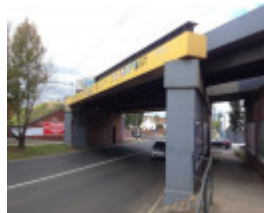
Rail over road bridge Ascot Vale Road
