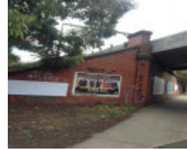
Rail over road bridge Ascot Vale Road
