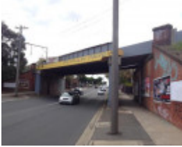
Rail over road bridge Ascot Vale Road
