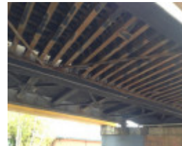
Rail over road bridge Ascot Vale Road
