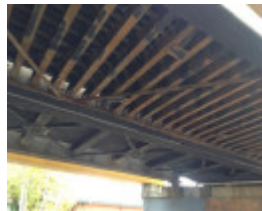
Rail over road bridge Ascot Vale Road
