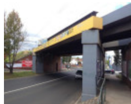
Rail over road bridge Ascot Vale Road
