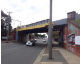
Rail over road bridge Ascot Vale Road
