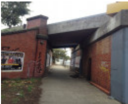
Rail over road bridge Ascot Vale Road
