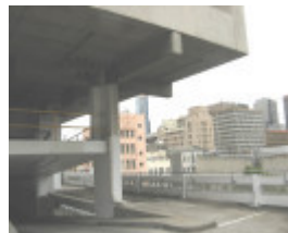
Total House office supports
