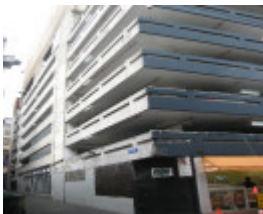
Total House laneway side
