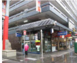
Total House corner shops
