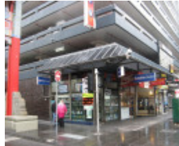
Total House corner shops
