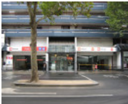
Total House Russell St entrance
