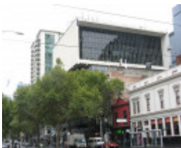
Total House view from south
