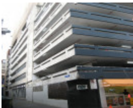
Total House laneway side
