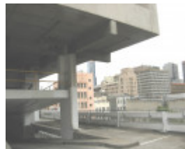
Total House office supports
