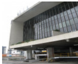
Total House office structure
