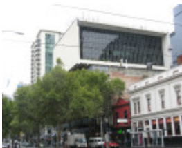
Total House view from south
