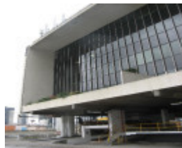
Total House office structure
