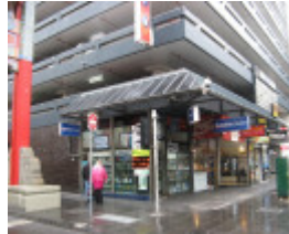
Total House corner shops
