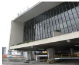
Total House office structure
