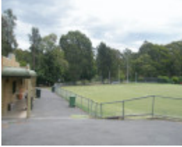
Former Memorial Park, 36 Greysharps Road, Hurstbridge
