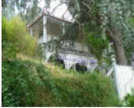
Residence, 760 Heidelberg-Kinglake Road, Hurstbridge
