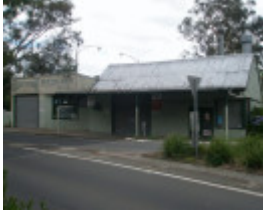
Garage, 849 Heidelberg-Kinglake Road, Hurstbridge, Front
