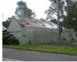
Garage, 849 Heidelberg-Kinglake Road, Hurstbridge, Rear
