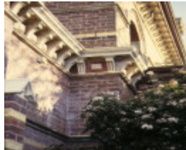
camperdown court house facade detail sep1997
