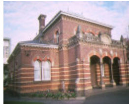
camperdown court house front elevation
