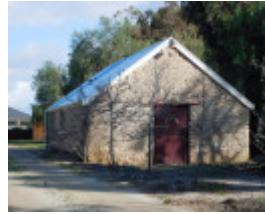
Laurence Park Stables repaired
