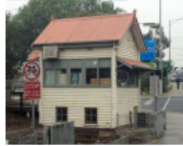
Gardiner railway signal box
