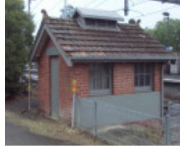
Gardiner switch house
