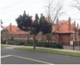
Former Infants School, Park Street.
