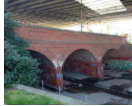
The east side of the bridge showing original 1891 brick arched construction.
