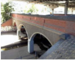
The west side of the bridge showing the 1912 addition.
