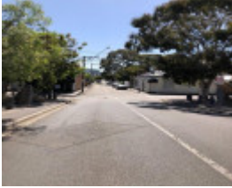
Argo Street Bridge
