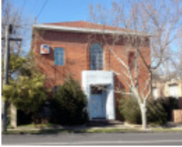
Toorak Telephone Exchange
