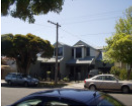
65-67 Maud Street, Geelong
