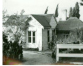
B2209 Moray Homestead Rear View
