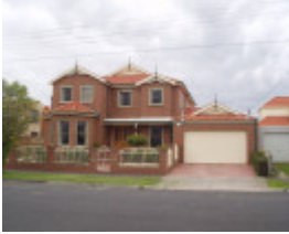
85 Maud Street, Geelong
