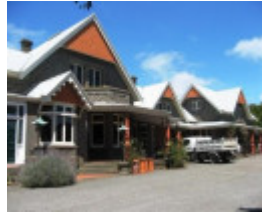
2013 North elevation of house
