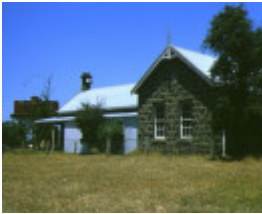
purrumbete camperdown bluestone building
