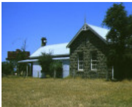
purrumbete camperdown bluestone building
