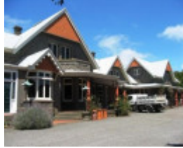
2013 North elevation of house
