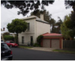
100 Maud Street, Geelong
