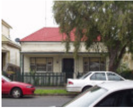
104 Maud Street, Geelong
