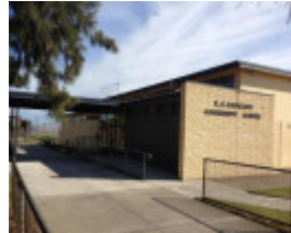
RG Ratcliff Community Centre
