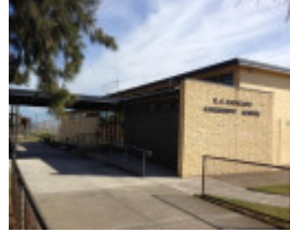
RG Ratcliff Community Centre
