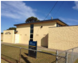
RG Ratcliff Community Centre
