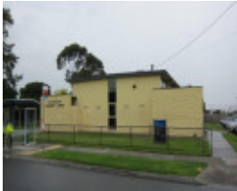
RG Ratcliff Community Centre
