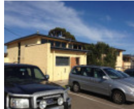
RG Ratcliff Community Centre
