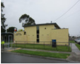
RG Ratcliff Community Centre
