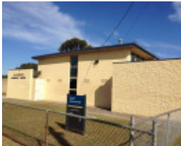
RG Ratcliff Community Centre
