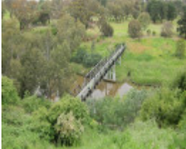
55 Canning Street, Avondale Heights (Maribyrnong River Pipe Bridge).JPG
