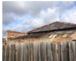
Aberfeldie House Stables
