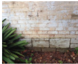
Aberfeldie House Stables
