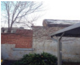
Aberfeldie House Stables
