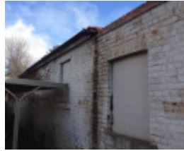
Aberfeldie House Stables
