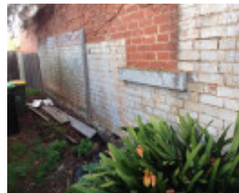
Aberfeldie House Stables
