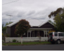
118 Maud Street, Geelong
