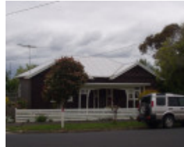
118 Maud Street, Geelong
