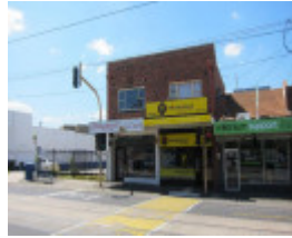
10-12 Keilor Road, Essendon
