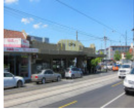
2 Keilor Road, Essendon
