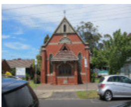
St Andrews Anglican Church, 29 St Kinnord Street, Aberfeldie
