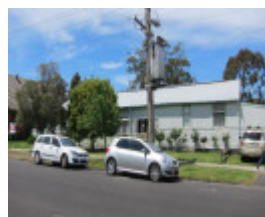
St Andrews Church Hall, 29 St Kinnord Street, Aberfeldie
