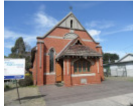
St Andrew's, facade
